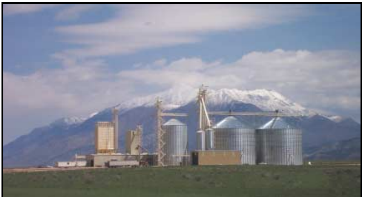
Taken from the south, this photo shows the combined IFA feed mill (left) and Moroni Feed Cooperative storage bins (right) near Nephi. The facility is capable of receiving a 100-car unit train of grain.
